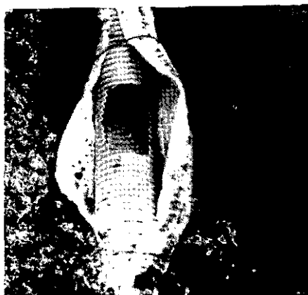
An exposed section of the pipe showing little evidence of silt.
