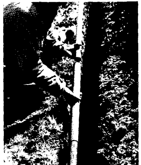
The junction of two 20 ft. lengths plastic pipe.
