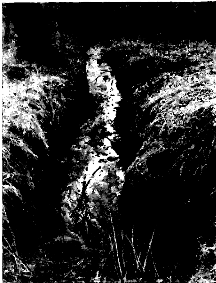
Ditch infilled with sediment.
