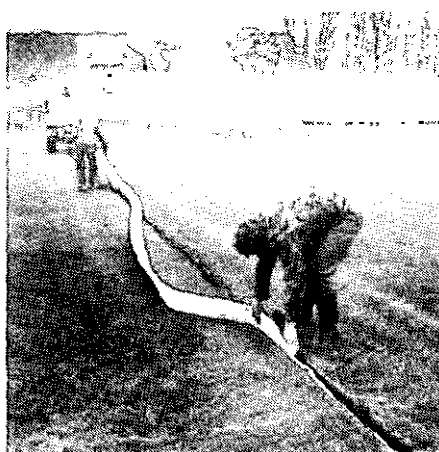
150mm HITEK STRIPDRAIN being laid at Melbourn Sports Stadium, Chelmsford
