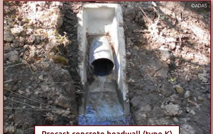
Precast concrete headwall (type K)
