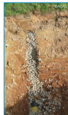
Permeable backfill in trench over drain
