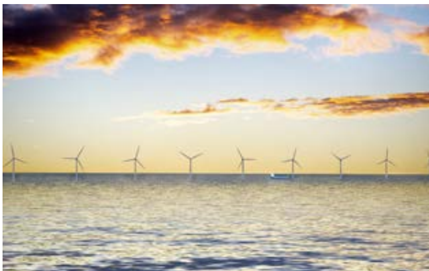
Currently 12 to 14MW turbine models with 220m rotors are typical offshore.
