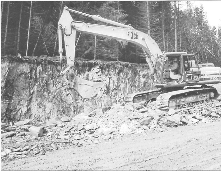
Fig. 5 Excavating rock adjacent to the roadline
