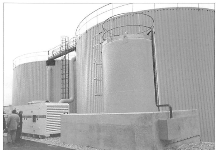
Surplus heated water, produced by the CHPs during the day, is stored in these tanks ready to be circulated through the glasshouses at night when the engines are not running. The tanks hold a total of 3,200 cubic metres and some idea of their size can be judged from the figures standing alongside.
