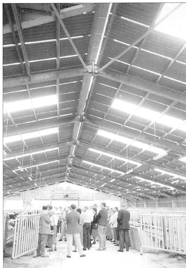
Fig. 4 Large livestock enterprises are housed in clear span structures with good light and ventilation. This one is designed for beef cattle, dairy young stock and pigs.
