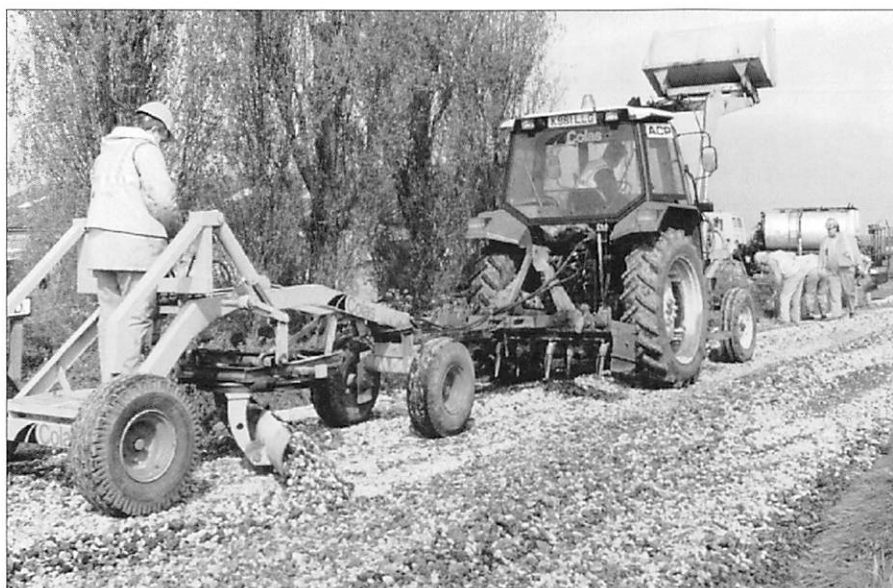
Fig. 5 Bitumen emulsion road rehabilitation using tractor technology [photo: Coles].
