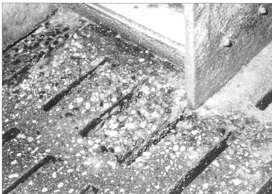
Fig. 1 Deterioration of concrete slats in front of a wetfeeder.
