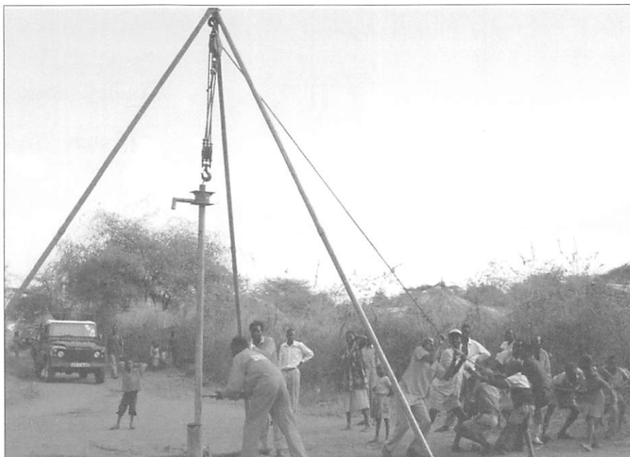
Fig. 4 Block and tackle system for lifting up 2 1/2 inch (64 mm) G.I. pipes.
