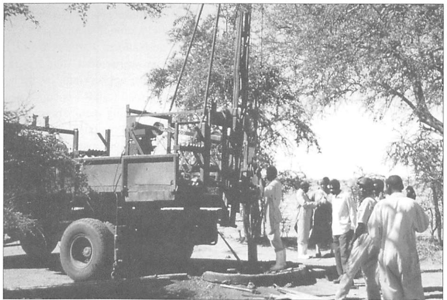
Fig. 1 Truck-mounted Dando 200 cable tool rig cleaning a borehole.
