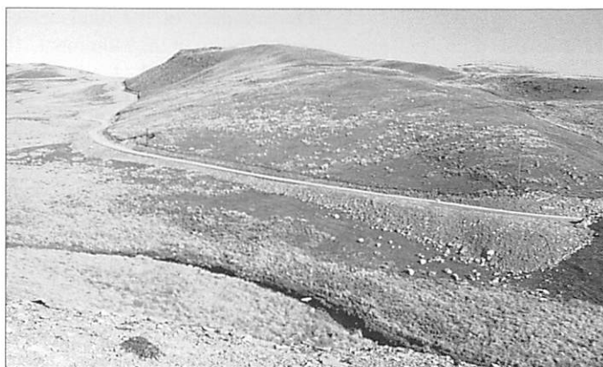
Fig. 9 Varying the road line in its horizontal and vertical dimensions achieves a sinuous, organic shape appropriate to this rounded, flowing landform
