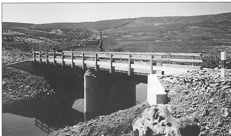
Fig. 3 Pollution free construction by means of a steel beam/timber deck bridge.
