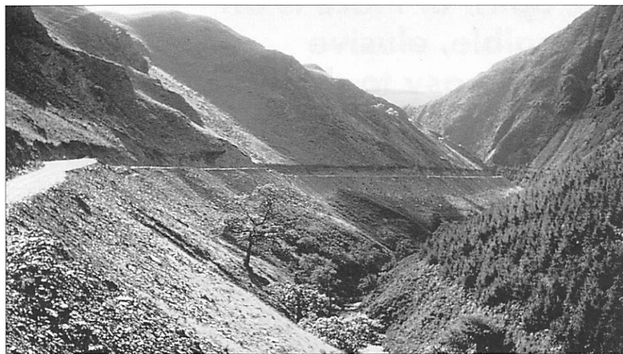
Fig. 7 This road, traversing a severe slope in rocky landform, results in a straight horizontal line and large amount of cut and fill which jointly contribute to its highly intrusive effect on this small to medium scale landscape.
