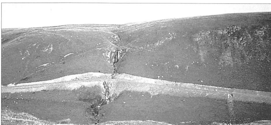
Fig. 10 Where roads cross open terrain in highly visible landscapes, avoid excessive excavations for cut and fill in light coloured materials which contrast strongly with surrounding vegetation
