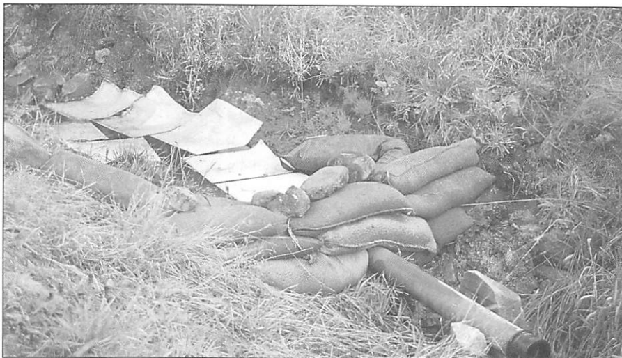
Fig.1 Absorbent pads in place behind a temporary dam.
