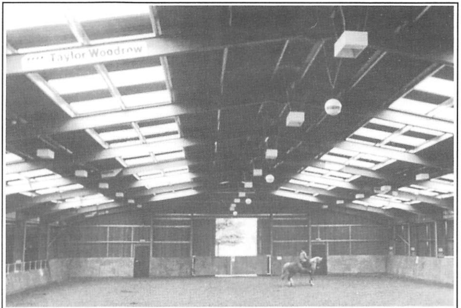
Wormwood Scrubs Pony Centre for the Handicapped using Filon G.R.P. sheets in a Chequer Board pattern resulting in no shadow at ground level. Material supplied in conjunction with the Anneka Rice Challenge.
