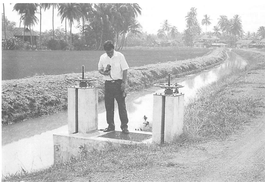
Constant Head Orifice (CHO) controlling the inflow into the tertiary canal.
