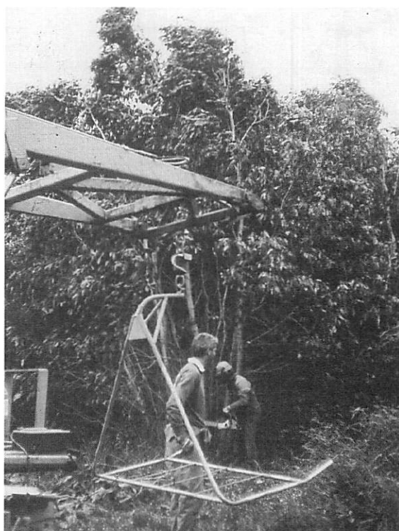
Fig 2. Motor manual harvesting of field experiments. The 3 year old coppice regrowth of the 9 year old Eucalyptus trees, being harvested for the third time, is weighed and recorded.
