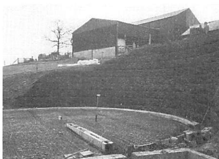
A 6m high earth wall constructed using Fortrac geotextile creates space for an effluent tank on Lancashire County Council's Smiths Farm.
