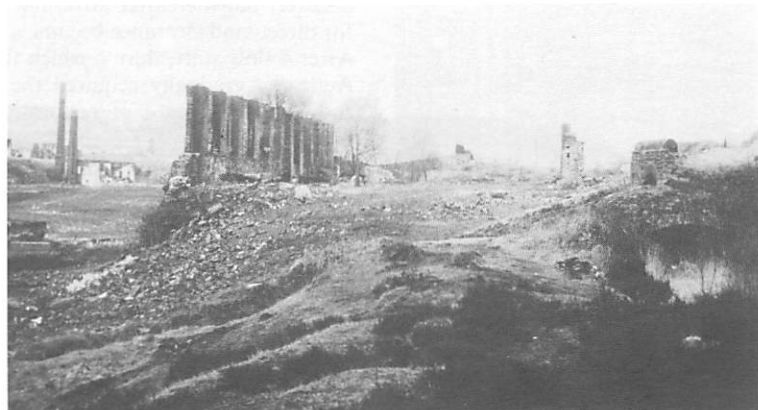
Remains of White Rock Works, Swansea.
