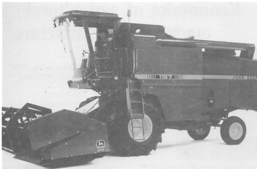
Fig 1. Component standardisation for cost reduction. Cabs and straw walkers are among standardised items in the John Deere range of combine harvesters.
