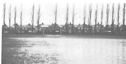
Water logged hard porous area due to fines and interlocking particles.
