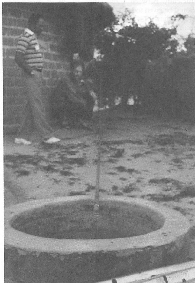
(a) Cover access-pit with gas supply pipe to the farmer's dwelling.
