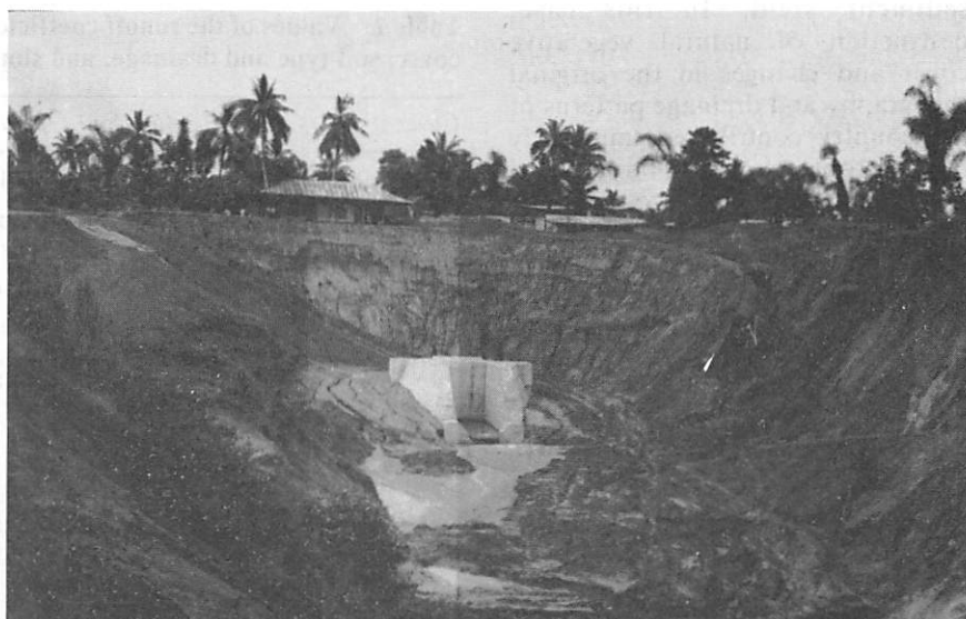
Fig 1 Slope stabilisation of gully endangering nearby houses
