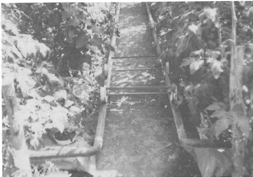
Fig 6 Lowering the heating pipes in a greenhouse improves the efficiency and as in this example from Wye College also enables the pipes to act as "rails" for material handling
