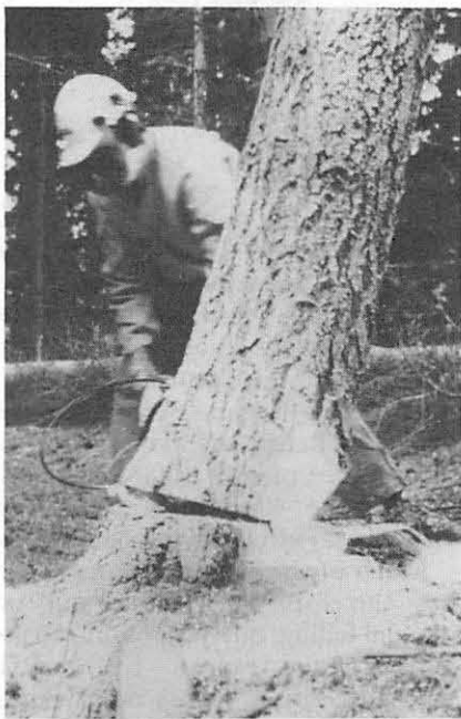
Fig 2 Felling using a Felling Cushion
