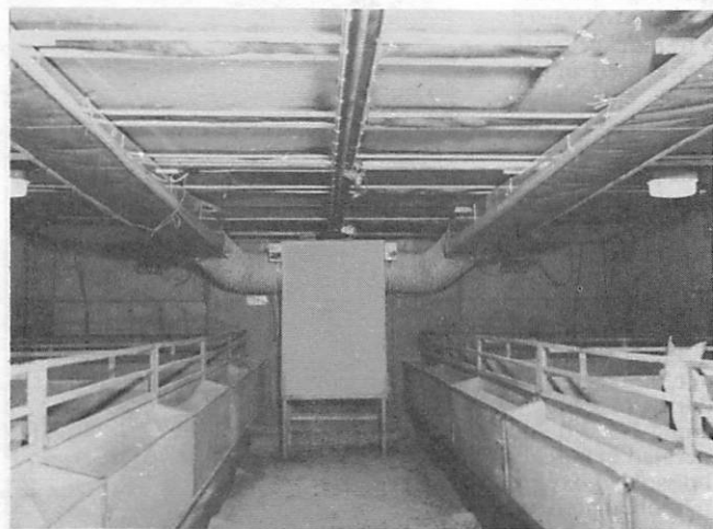
Fig 1 Experimental dust filter (NIAE photo)
