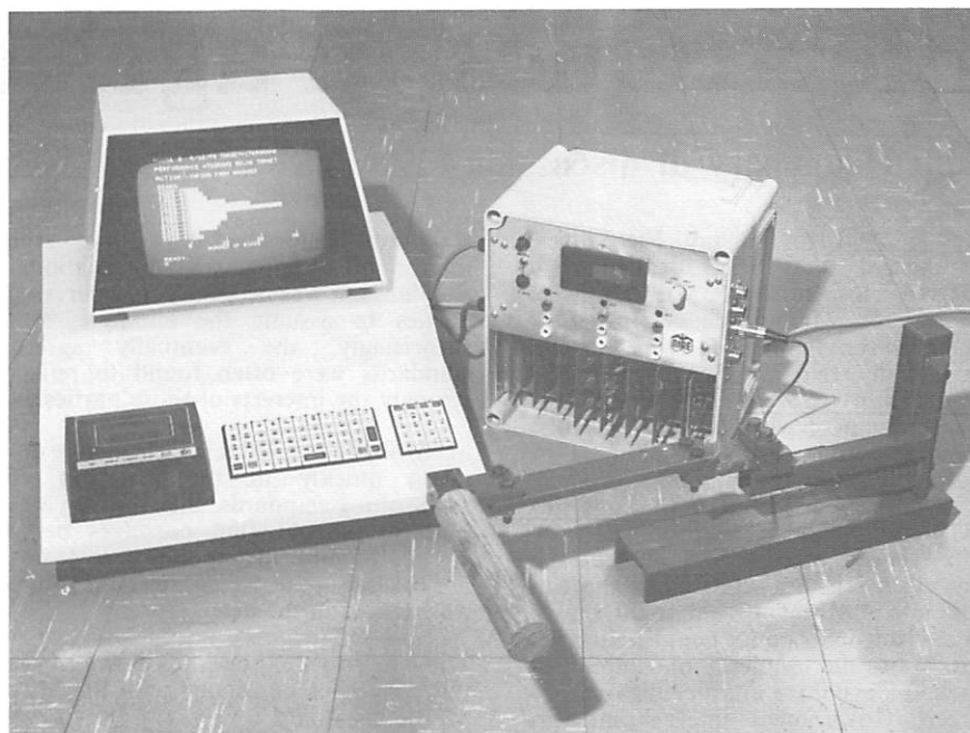
Fig 2 Personal computer applied to monitoring of broiler weights Foreground — strain gauged perch Background — signal conditioning unit
