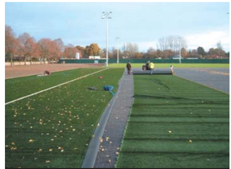
NOVEMBER 2007 Laying synthetic carpet on all-weather pitch
