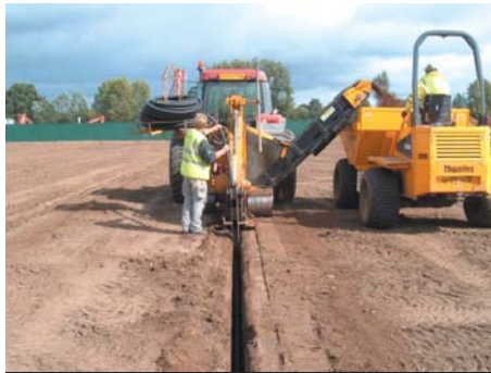
SEPTEMBER 2007 Drainage installation on match pitch
