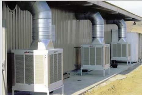
An evaporative cooling system: the ideal solution for beating the heat in agricultural storage and livestock facilities during summer, as it reduces temperatures by up to five times that of ventilation alone
