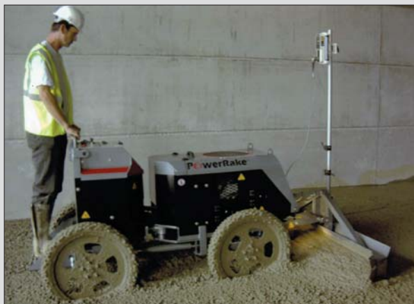
PowerRake is a one-man laser controlled four-wheel drive ride-on raking system which delivers better results in less time
