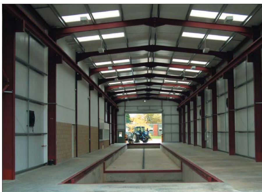
Fig.3 New 45 m long, 5 m wide soil lane (shown empty prior to soil fill)
