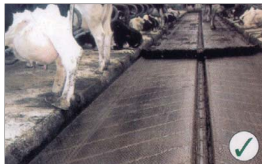
Example images: steps down giving an injury risk; well-drained herringbone floor
