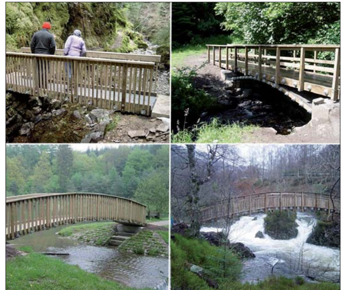
Fig. 12 Example of stress laminated timber bridges: 5 m span flat deck Pucks Glen (top left); 9 m arch and flat deck at Stewarton (top right); 9 m span Mallards Pike (bottom left); 17 m span Achray (bottom right)
