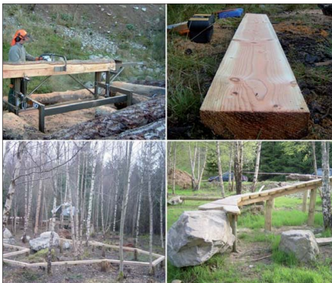
Fig. 4 Construction of skinny structure: bench saw (top left); skinny top log (top right); longitudinal logs (bottom left); and skinny runway constructed using skinny top logs fixed to the longitudinal logs (bottom right)
