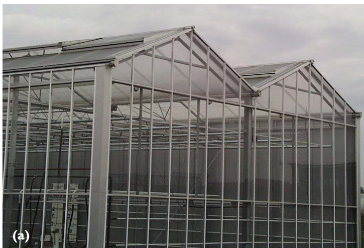
(a) First greenhouse with extruded zigzag sheets of Lexan® Zig Zag™ in Elst, Netherlands; and (b) detail of the roof construction with the extruded zigzag sheets
