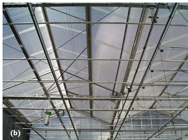
(a) First greenhouse with extruded zigzag sheets of Lexan® Zig Zag™ in Elst, Netherlands; and (b) detail of the roof construction with the extruded zigzag sheets
