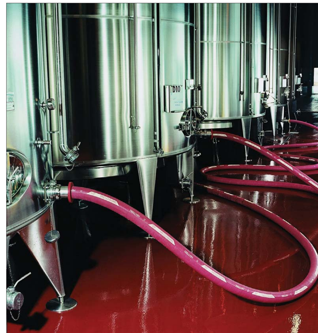
Hoses that transport wines must meet stringent hygiene requirements, so all Trelleborg's hoses are equipped with the white, smooth inner lining that prevents impurities and bacteria from gaining hold and guarantees cleaning with perfect results.
