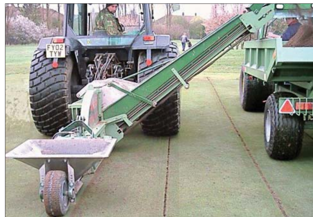
Shelton System 25 draining an established golf green; trenches are 25 mm wide and are simultaneously being backfilled with Lytag
