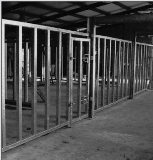
Galvanized steelwork forming part of the new Rhino House at Flamingo Land Theme Park and Zoo
