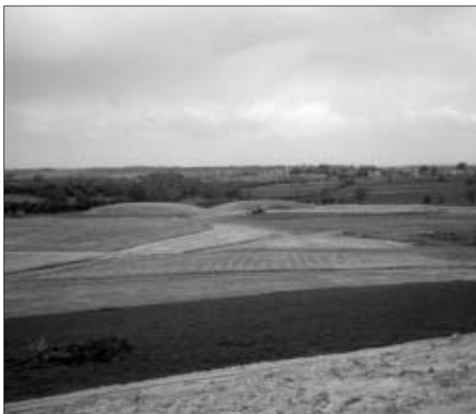
Landscape view of an opencast site showing, from the left, re-instated topsoil, subsoil and overburden horizons. In the background, storage bunds and settlement lagoons can be seen
