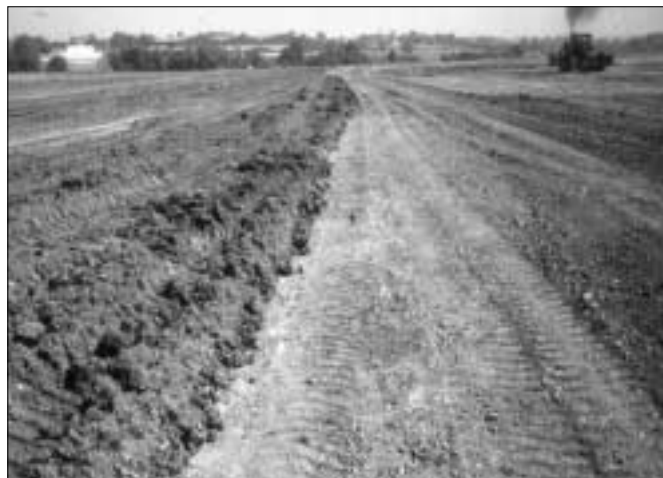
Re-instated sub and topsoil layers in close-up. Drainage and deep ripping is required to provide hydraulic connection between these layers, but this will ultimately fail unless the biological community is properly managed to stabilise and develop an open soil structure
