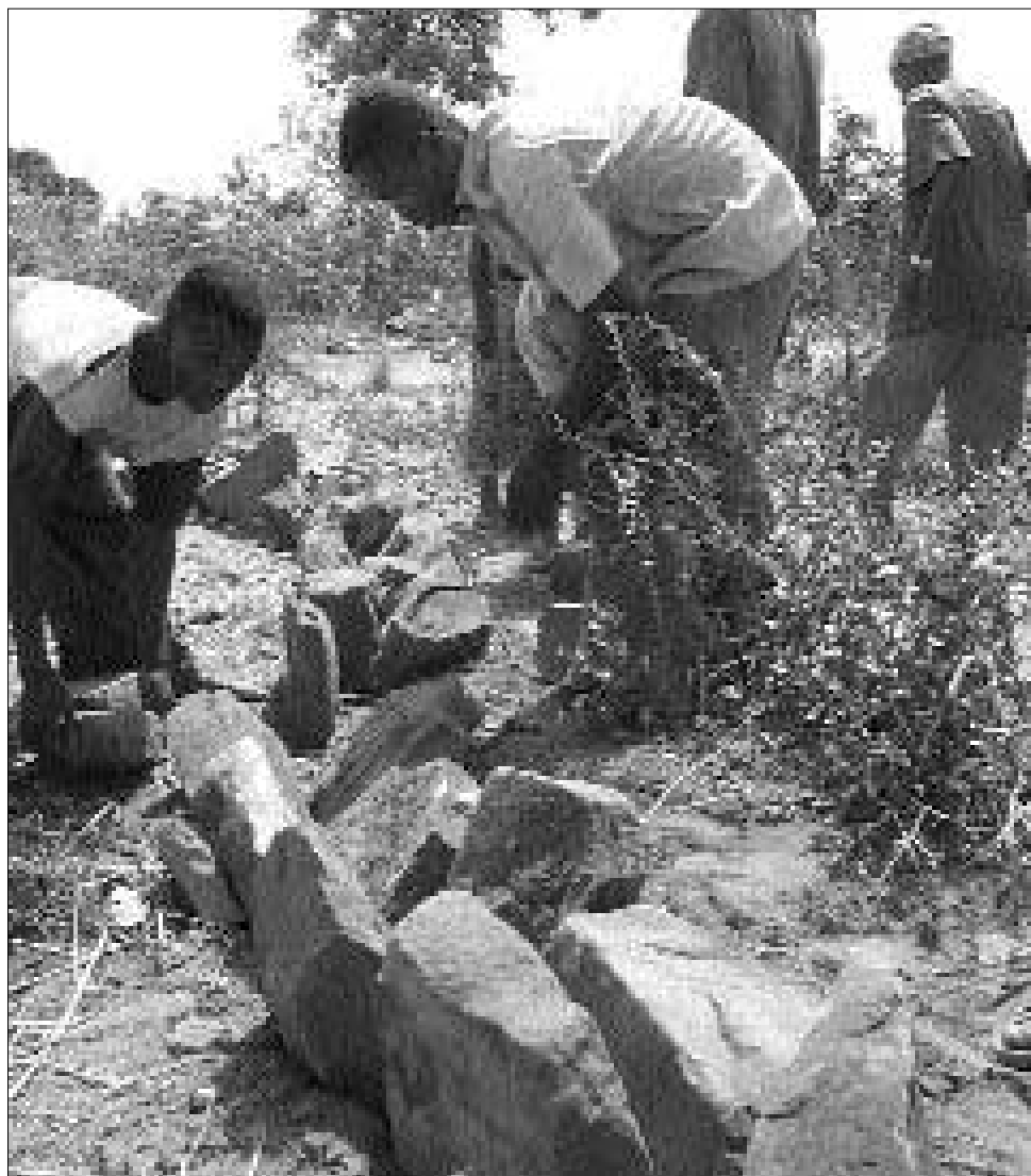
Farmers laying the foundations of a new stone bund
