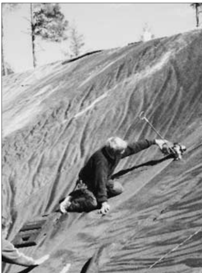
Seam welding of the 90 m x 5 m panels with an automatic seam-welding device producing channel welds
