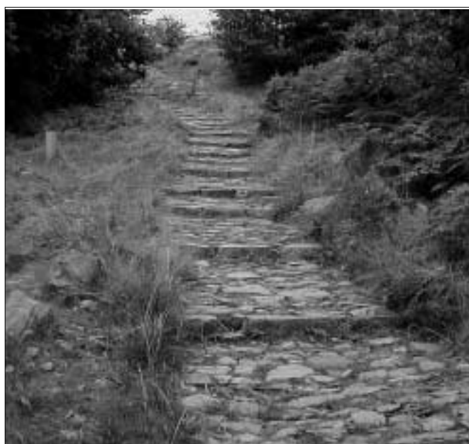
This finished path at Orrest Head in Cumbria has a hardwearing surface that carries over 100,000 people per annum; it has excellent revegetation, giving a natural appearance and was built in the same style as the Inca trail, Peru (Photo: Andy Carling)
