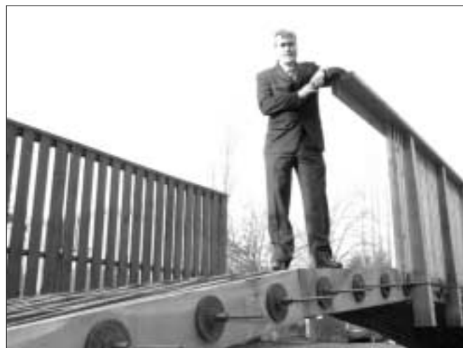
Scottish Minister for Enterprise, Transport and Lifelong Learning, Iain Gray, crossing Geoff Freedman's novel bridge design in stress laminated timber after opening the Centre for Timber Engineering at Napier University
