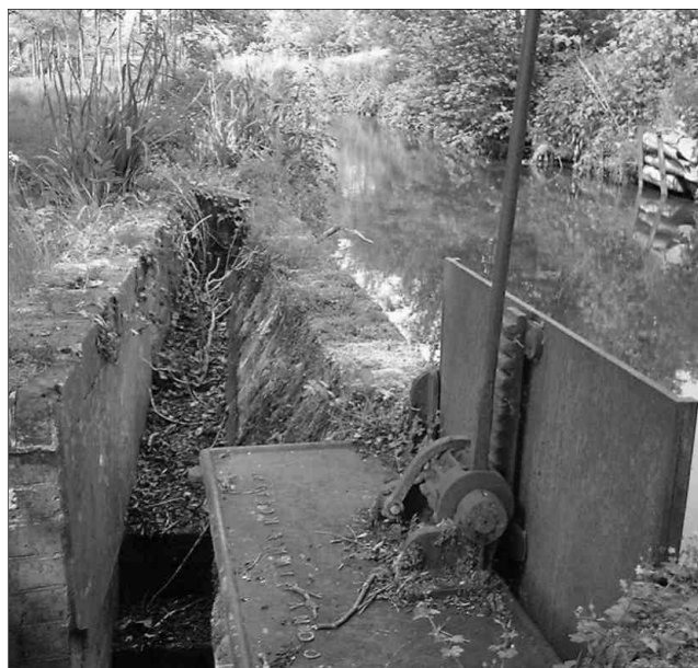
Iron sluice with brickwork overflow in Test Valley - Grid Ref. SU 479481
