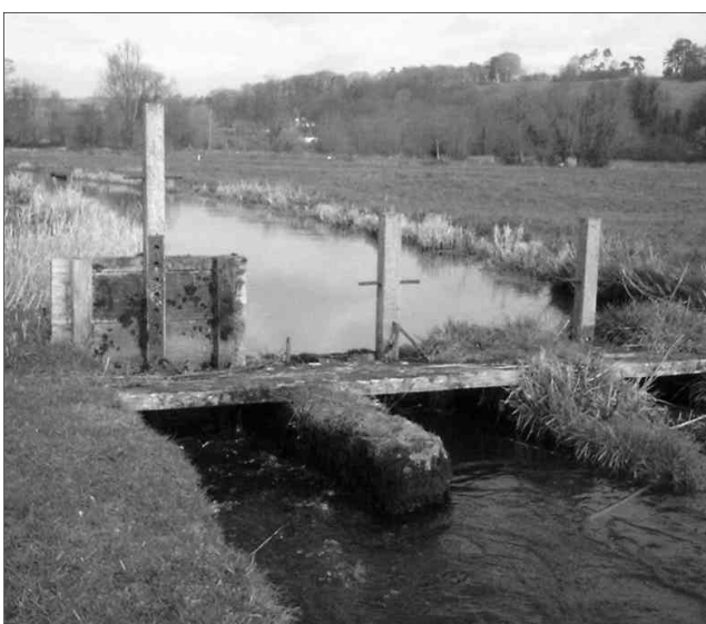
Stone sluice with wooden boards – Avon Valley Grid Ref. SU 125352
