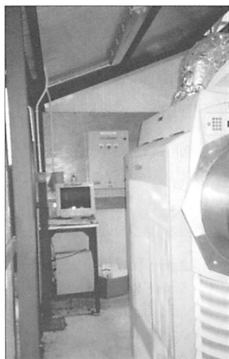
Computer controlled, the Minigen unit is relatively small. The air inlet is seen centre right and the insulated exhaust top right
