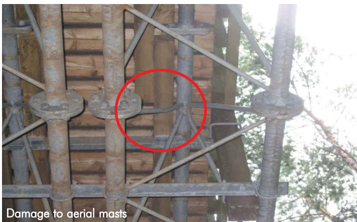
Loose bolts in tower bracing
