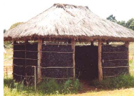
Fig.4: A passive cooler with charcoal walls. Note how the charcoal has settled to give a gap above and the fact that weeds have grown up to partially obstruct airflow
