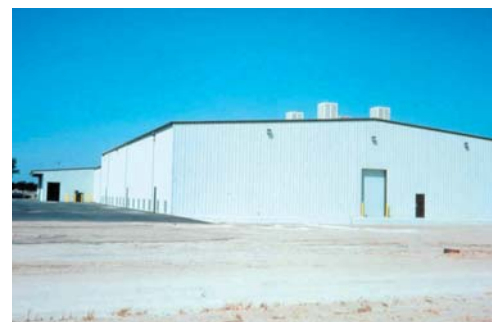
Fig.3: A 10,000t store in California with the cooler units on the roof and pressure flaps on the side
