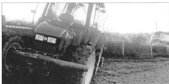
Vulcan high tensile stockfence from Tinsley Wire being erected for Great Western Railways
