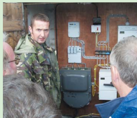
Eoin showing where 3 phase power enters and leaves the farm
