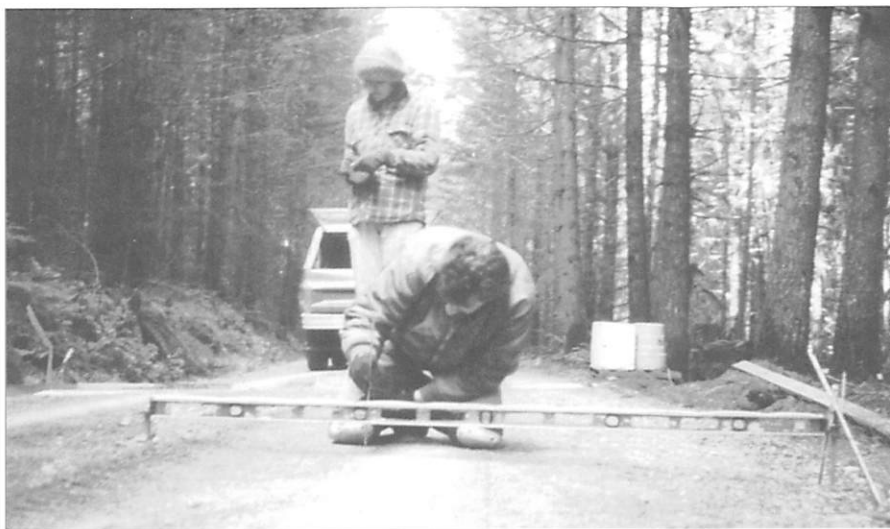
Fig. 2 Measuring rutting on a road in the Willamette National Forest, OR.
