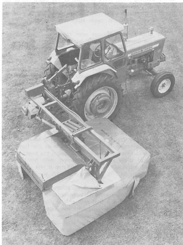
Fig 5 NIAE experimental mower-conditioner with improved guarding.
