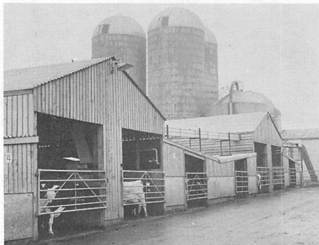
A view of Bridget's EHF showing the cow houses and overhead conveyors carrying mixed rations to groups of animals. The weighing and automatic control equipment is in the building in the background.
