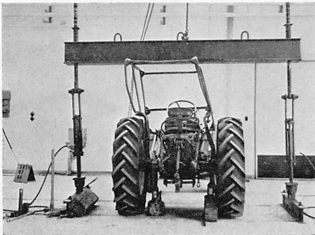
FIG. 4. Crushing Test at Swedish Testing Station for Agricultural Machinery (Alnarp)
