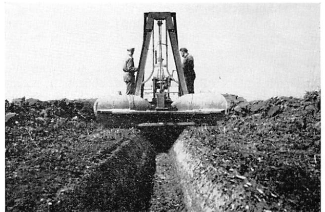
Trenching plough. Trenches are 1.15 metres wide, 60 c.m. deep and 25 c.m. in the bottom; content, 0.42 cubic metre.
