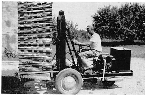
FIG. 4. A home-made fork-lift truck designed and built by a Canadian fruit grower.
