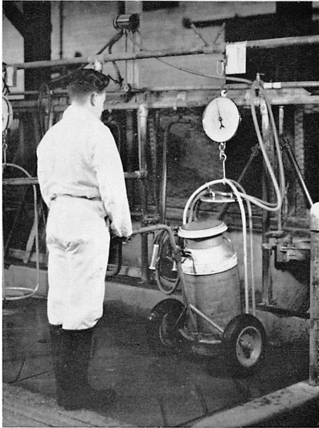
Fig. 5. The simple method of moving full cans of milk from the milking point in a direct-to-can parlour.
