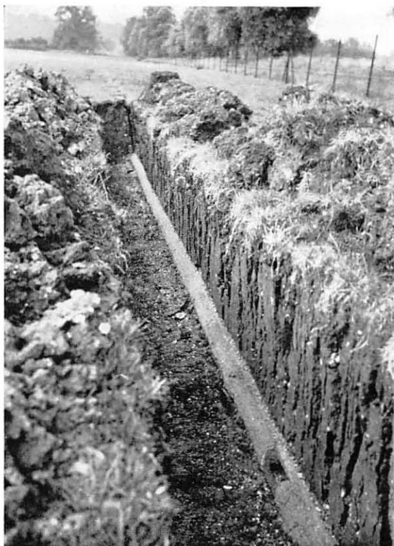
FIG. 8.—Excavated Section of Tube Laid in Gault Clay.
