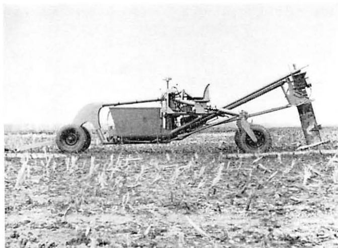
FIG. 6.—Vibration System Mole Plough as first fitted for Extensive Fieldwork.
